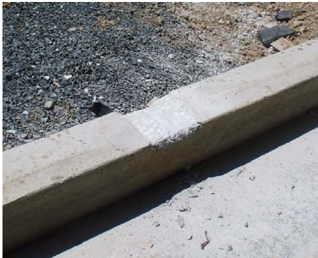
Concrete Curb Chip-Out Ground Floor
