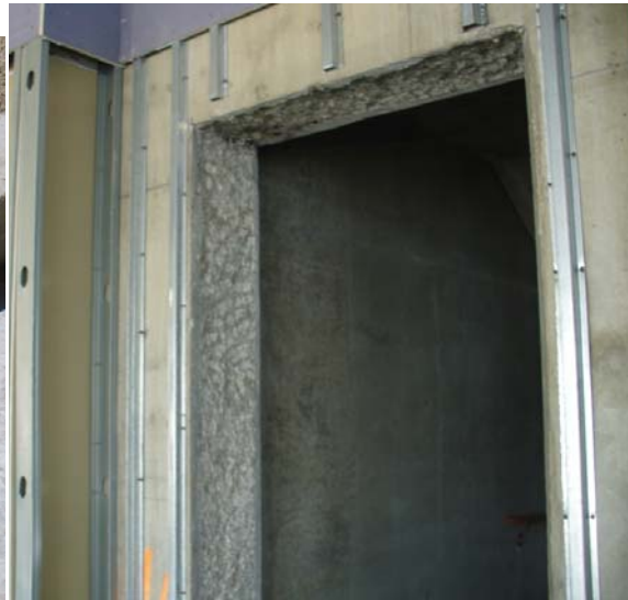
Concrete Door Chip-Out
